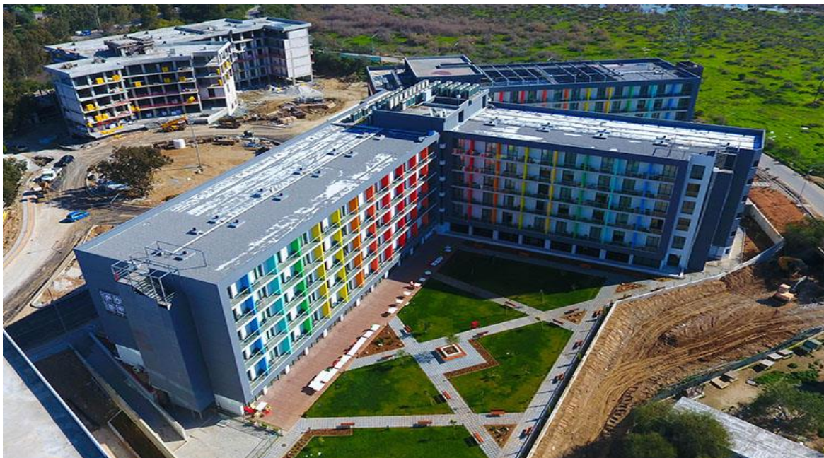
Fig 4: Western and Northern façade of the building in which shading devices are absence (Neden Mağusa'da Pop Art Öğrenci)
