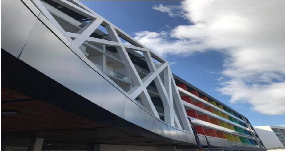
Fig 3: Showing the X shape shading devices on the eastern Façade (Faisal Saleh Minangi Archive,2018)
